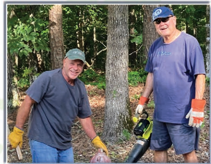
Doug and Greg clearing the ground
